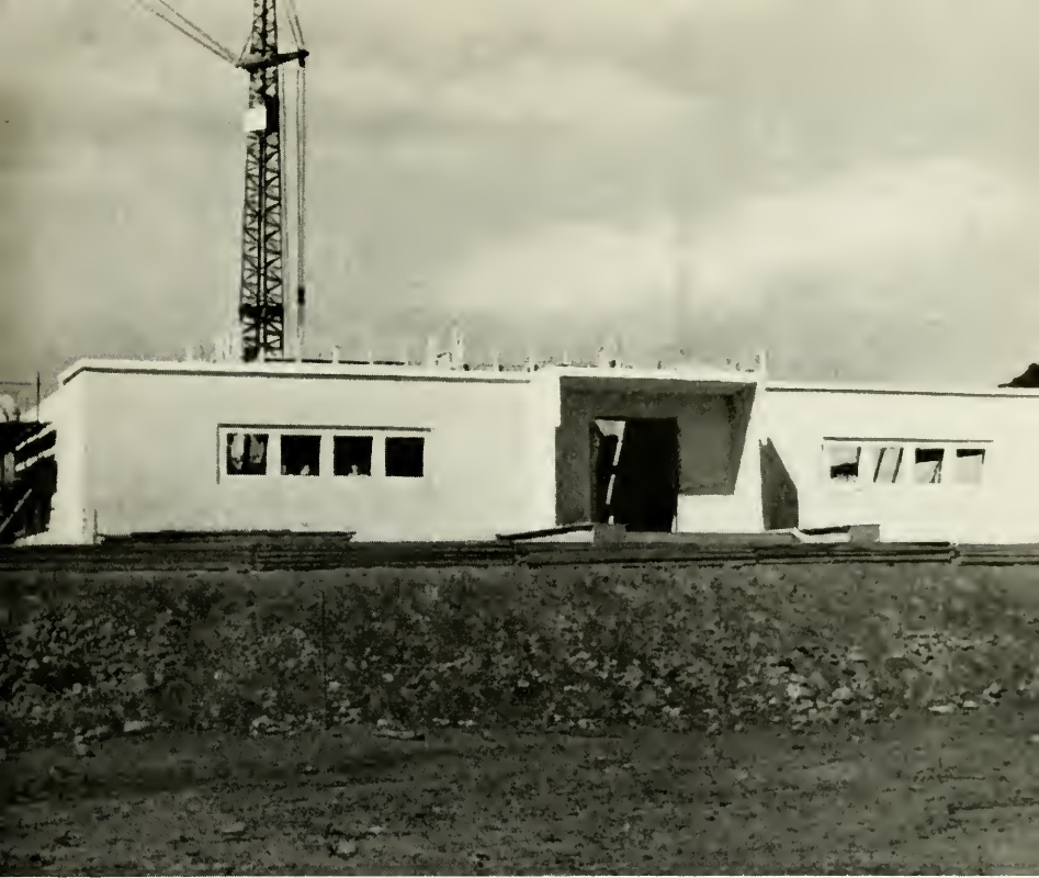
Progress in May, 1957
